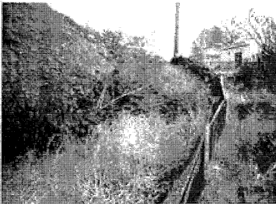
Silt fence not installed on contour
