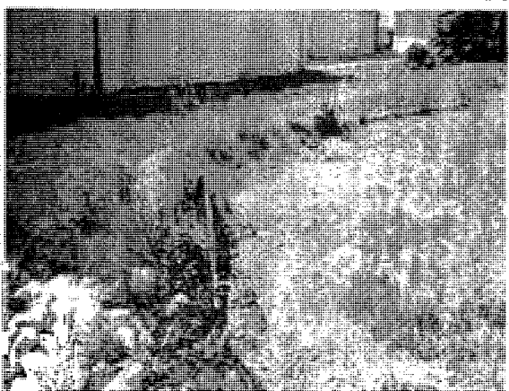
Compost filter sock maintained in place at Sediment Basin 1
