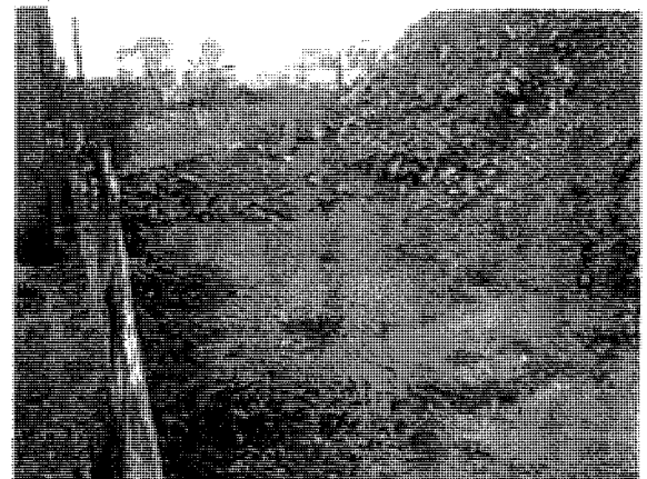
Sediment eroding off side slope of unstabilized fill
