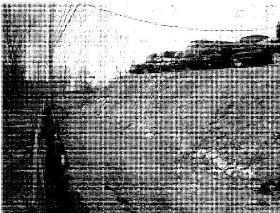
Compost filter sock installed downslope of fill slope
