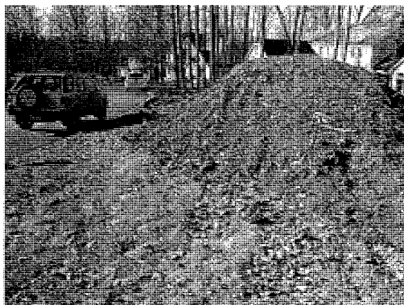
Compost filter sock not entirely downslope of stockpile
