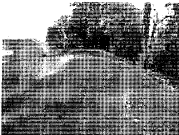
Top of berm and super silt fence
