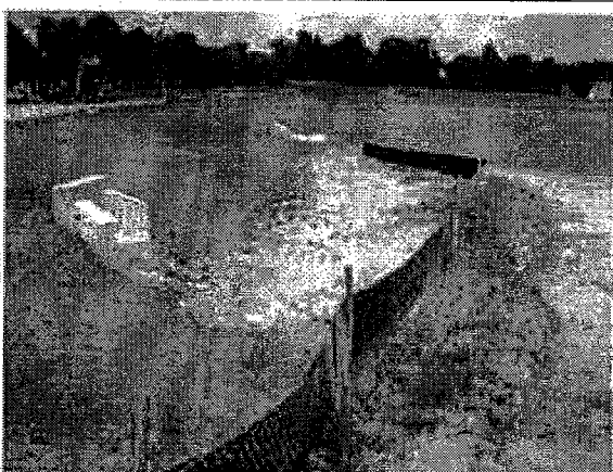
Sediment Trap 1 baffle
