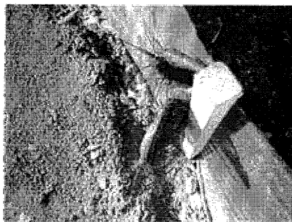
Silt fence joints not wrapped watertight
