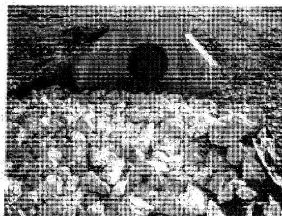
Basin converted with rock lined low flow channel installed
