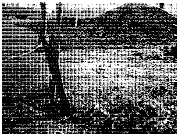
Compost filter sock not entirely downslope of stockpile or earth disturbance and sediment deposited outside LOD
