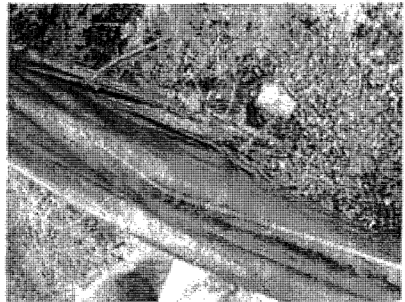
Silt fence not trenched in along bottom edge of fabric
