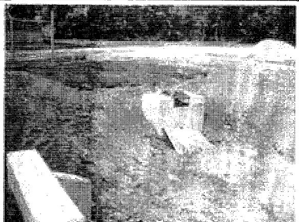
Rain Garden #2 emergency spillway lined
