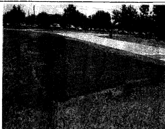
Sediment Trap 1 emergency spillway lined
