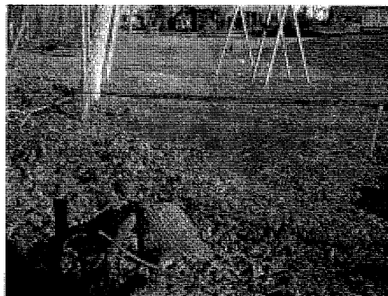
Compost filter sock not entirely downslope of stockpile or earth disturbance and sediment deposited outside LOD
