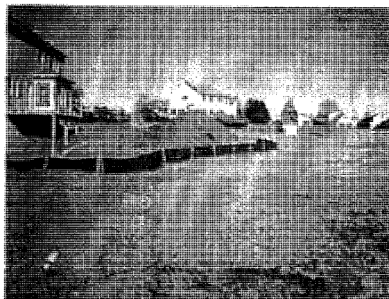
Silt fence not installed downslope of all areas of earth disturbance
