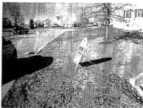
Lot 59 under construction with no silt sacks in nearest inlets
