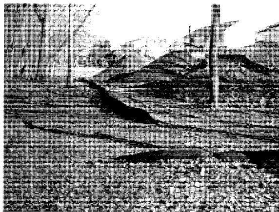
Gap in compost filter sock at NW corner of LOD
