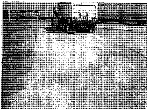
Rock construction entrance maintained
