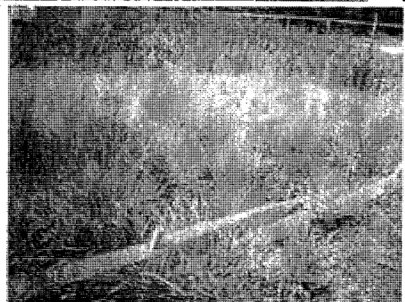
Compost filter sock maintained in place along south east perimeter
