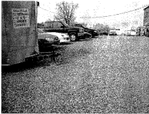
Rolled stone applied to parking area
