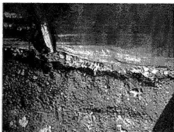
Silt fence not trenched in along bottom of fabric
