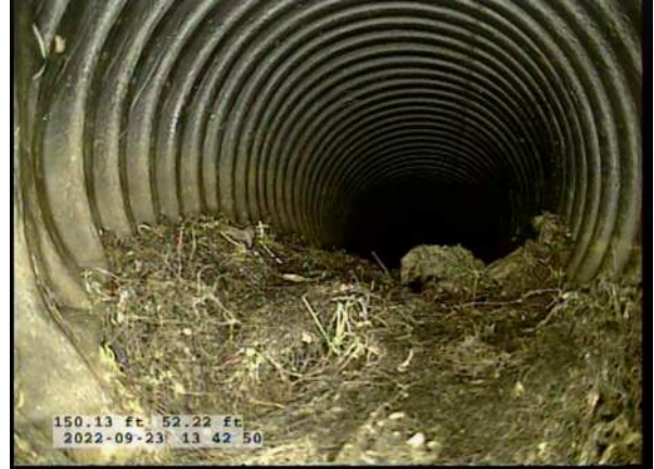
10, 00:03:31, 49.30ft Roots Medium Barrell from 5 o'clock to 7 o'clock, 10% of cross sectional area, Start
