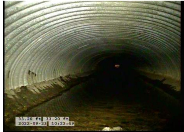
6, 00:02:14, 33.20ft Water Level, 10% of the vertical dimension
