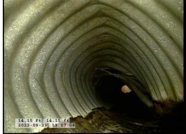
10, 00:02:29, 14.15ft Miscellaneous General Observation / DAYLIGHT AT CB4 VISIBLE
