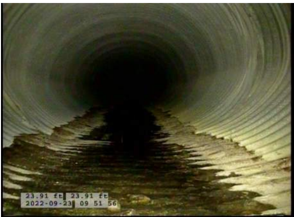
7, 00:01:22, 23.91ft Deposits Settled Compacted, 5% of cross sectional area at 6 o'clock, within 8 inch, Finish
