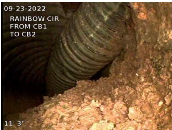
7, 00:00:56, 11.25ft Miscellaneous General Observation / 10 INCH CPP PIPE FROM CB2 VISIBLE
