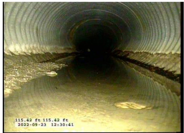
12, 00:09:54, 115.42ft Water Level, 5% of the vertical dimension
