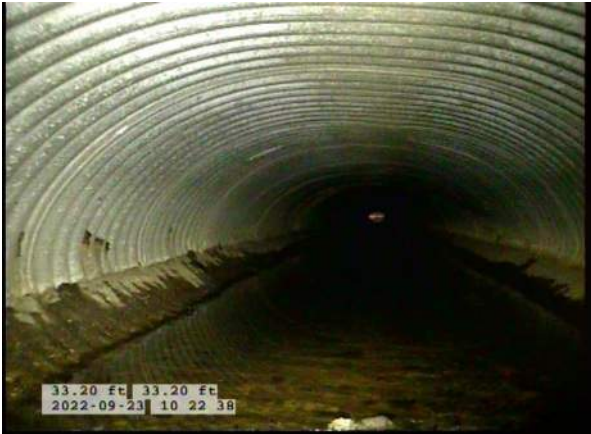
5, 00:02:12, 33.20ft Deposits Settled Gravel, 5% of cross sectional area from 6 o'clock to 7 o'clock, within 8 inch, Finish
