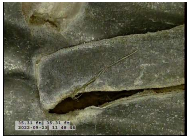
12, 00:04:04, 35.31ft Hole Soil Visible from 2 o'clock to 3 o'clock
