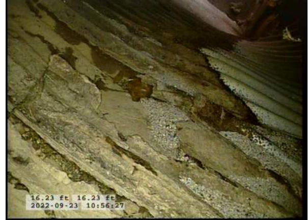
6, 00:01:53, 16.23ft Surface Damage Missing Wall from 5 o'clock to 7 o'clock / BOTTOM OF PIPE RUSTING AWAY
