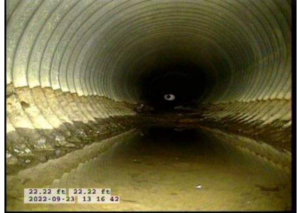
6, 00:02:43, 22.22ft Water Level, 5% of the vertical dimension
