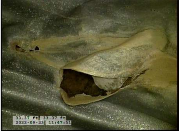
9, 00:03:28, 33.37ft Hole Soil Visible from 2 o'clock to 3 o'clock
