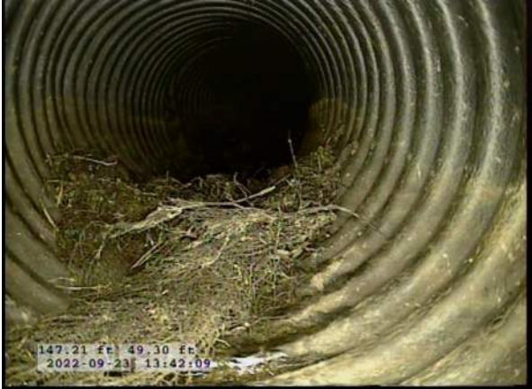
9, 00:03:31, 49.30ft Roots Medium Barrell from 5 o'clock to 7 o'clock, 10% of cross sectional area, Start
