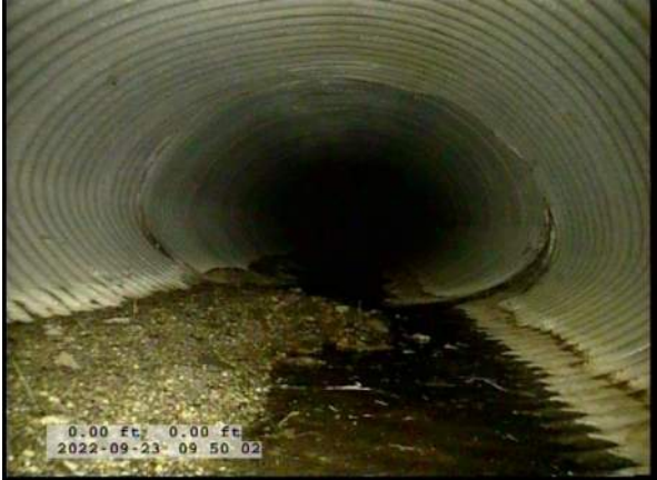
1, 00:00:10, 0.00ft Catch Basin / CB11
