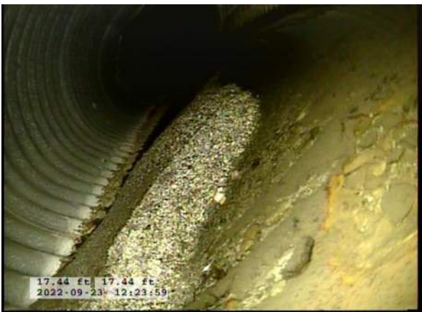
11, 00:03:18, 17.44ft Deposits Settled Fine, 5% of cross sectional area from 6 o'clock to 7 o'clock
