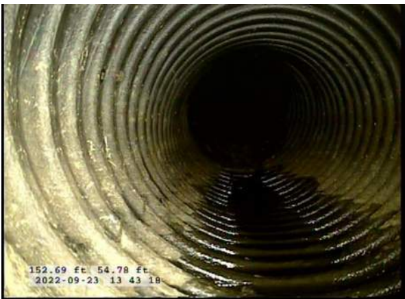
11, 00:04:32, 54.78ft Roots Medium Barrell from 5 o'clock to 7 o'clock, 10% of cross sectional area, Finish
