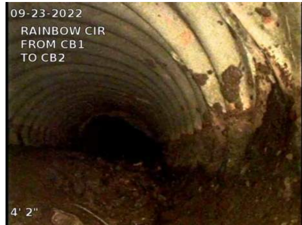
6, 00:00:19, 2.16ft Deposits Settled Gravel, 10% of cross sectional area from 5 o'clock to 7 o'clock, within 8 inch, Start
