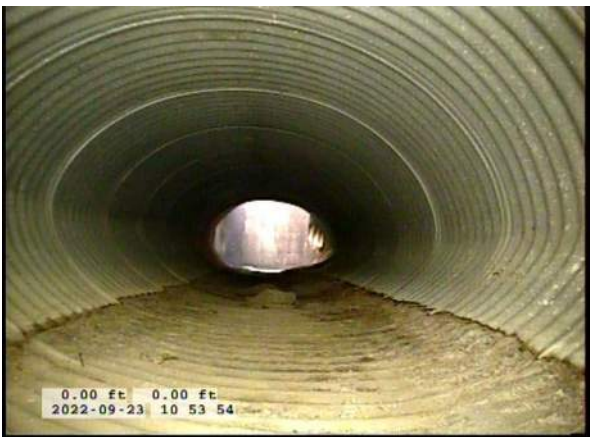
3, 00:00:16, 0.00ft Deposits Attached Encrustation, 5% of cross sectional area from 5 o'clock to 7 o'clock, within 8 inch, Start
