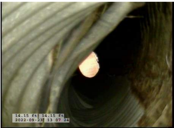
11, 00:02:29, 14.15ft Miscellaneous General Observation / DAYLIGHT AT CB4 VISIBLE
