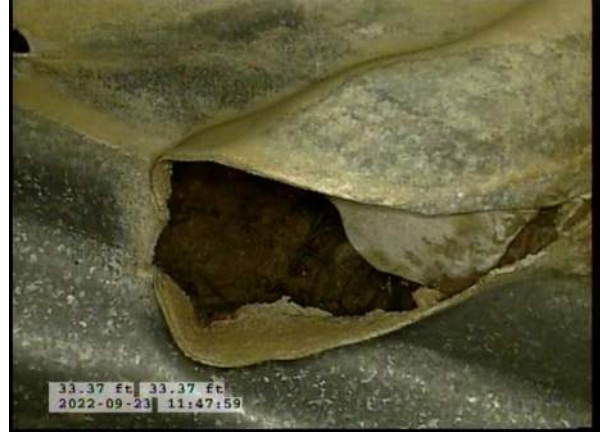
10, 00:03:28, 33.37ft Hole Soil Visible from 2 o'clock to 3 o'clock
