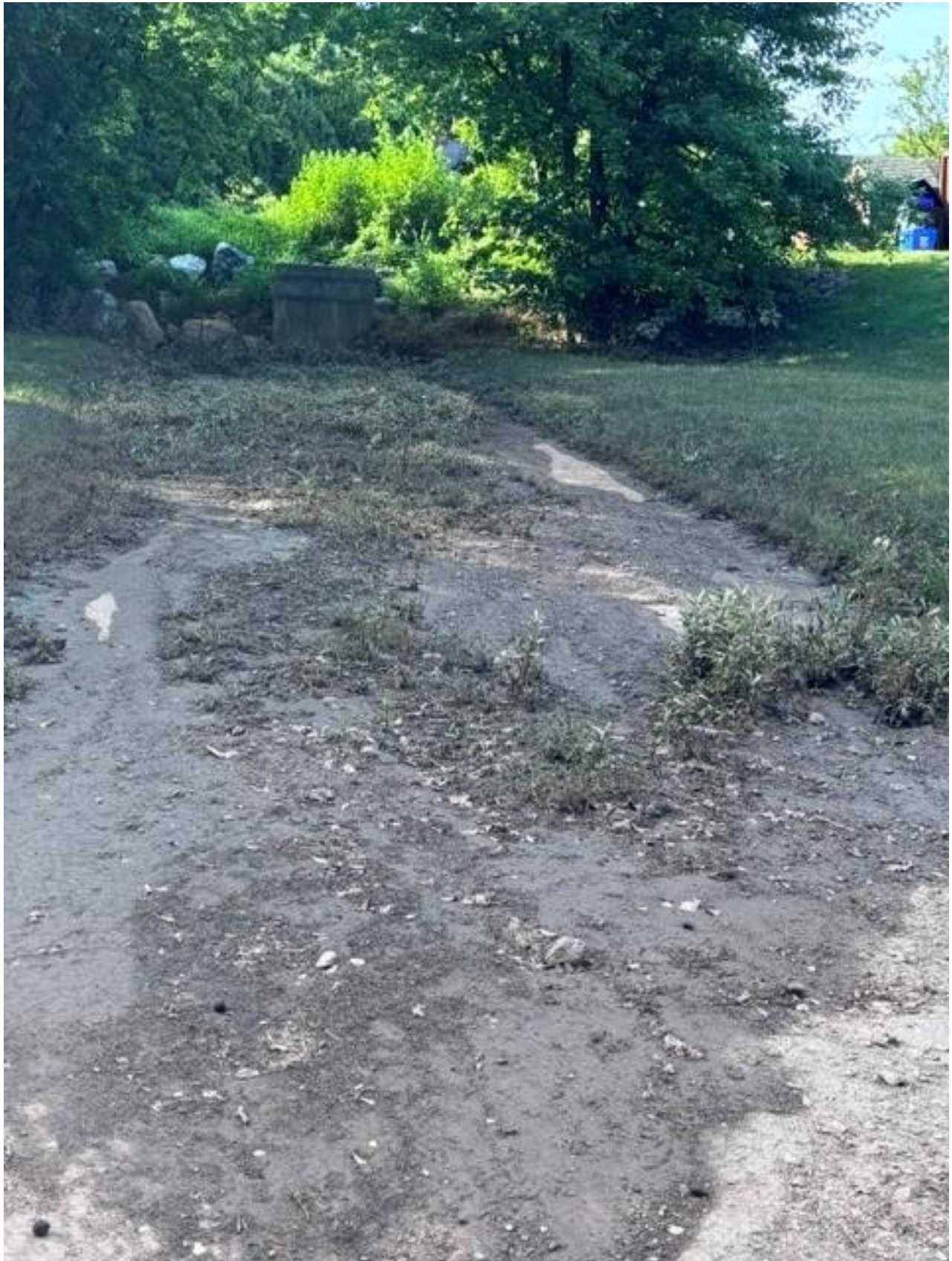
Weldon Rd Storm Water After
