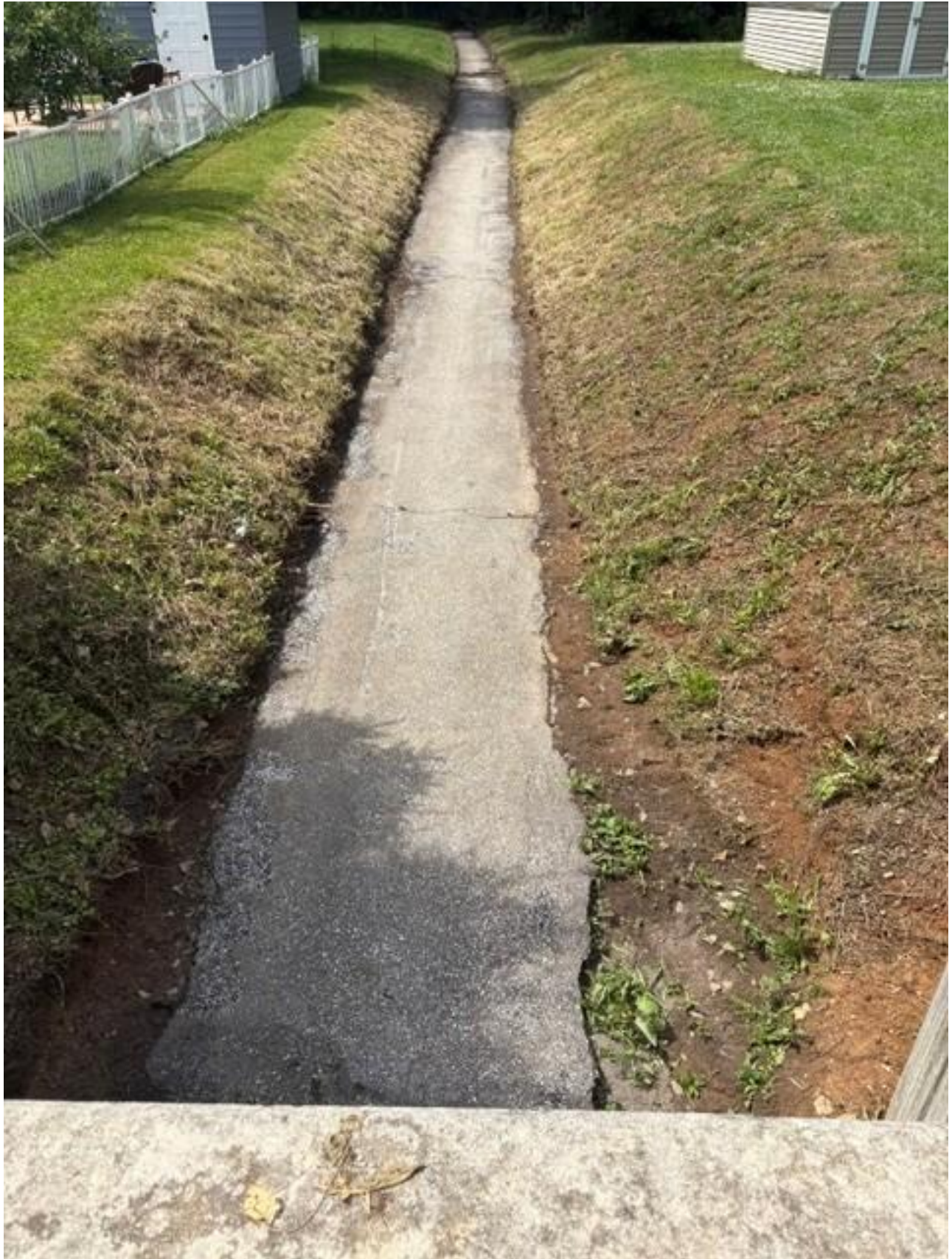
AFTER - HESS RD
