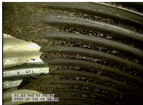
8, 00:03:14, 91.43ft Miscellaneous General Observation / BITUMINOUS COATING ON THIS LENGTH OF THE PIPE
