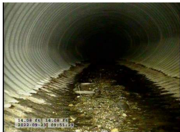
6, 00:00:59, 14.08ft Deposits Settled Compacted, 5% of cross sectional area at 6 o'clock, within 8 inch, Start
