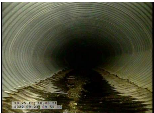
5, 00:00:44, 10.25ft Deposits Attached Encrustation, 5% of cross sectional area from 5 o'clock to 7 o'clock, within 8 inch, Start / RUST
