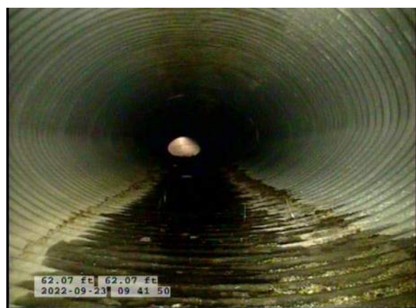
8, 00:03:37, 62.07ft Deposits Settled Gravel, 5% of cross sectional area from 5 o'clock to 7 o'clock, within 8 inch, Finish
