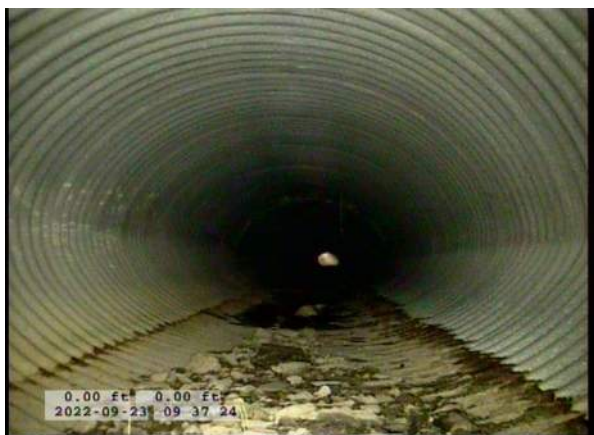
1, 00:00:09, 0.00ft Catch Basin / CB11
