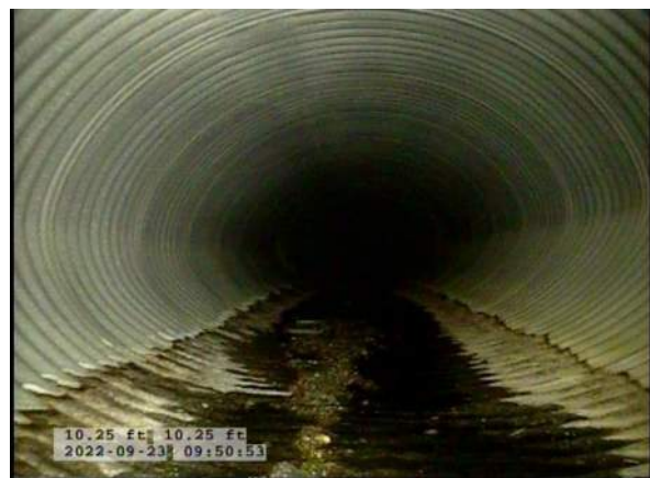
4, 00:00:42, 10.25ft Deposits Settled Compacted, 5% of cross sectional area from 6 o'clock to 7 o'clock, within 8 inch, Finish
