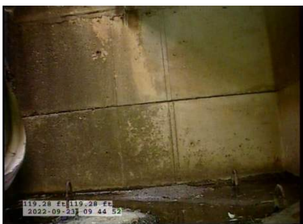
11, 00:06:07, 119.27ft Deposits Settled Gravel, 5% of cross sectional area from 5 o'clock to 7 o'clock, within 8 inch, Finish
