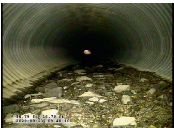
7, 00:02:00, 16.79ft Deposits Settled Gravel, 5% of cross sectional area from 5 o'clock to 7 o'clock, within 8 inch, Start
