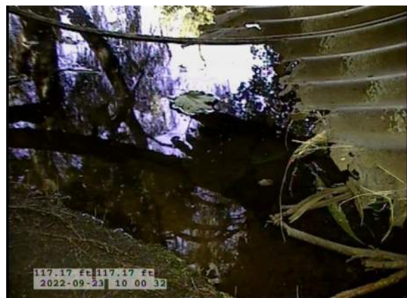
14, 00:07:26, 117.17ft Miscellaneous General Photograph from 5 o'clock to 7 o'clock / BOTTOM OF PIPE COMPLETELY MISSING AT END OF PIPE
