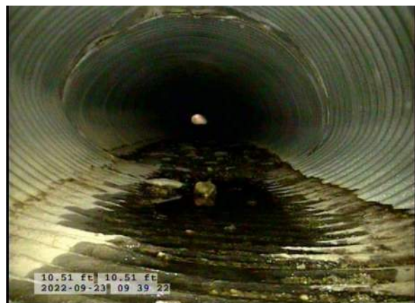
6, 00:01:21, 10.51ft Deposits Settled Gravel, 5% of cross sectional area at 6 o'clock, within 8 inch, Finish
