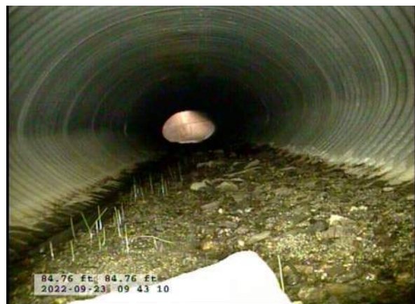
10, 00:04:32, 84.76ft Deposits Settled Gravel, 5% of cross sectional area from 5 o'clock to 7 o'clock, within 8 inch, Start
