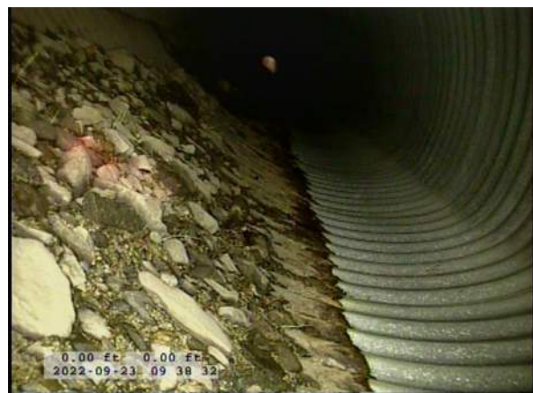
4, 00:00:34, 0.00ft Deposits Attached Encrustation, 5% of cross sectional area from 5 o'clock to 7 o'clock, within 8 inch, Start / RUST
