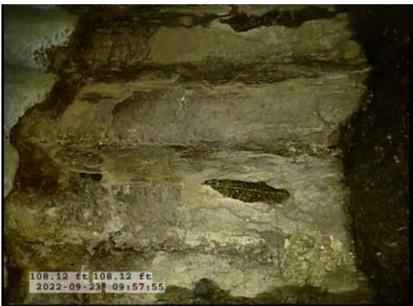
11, 00:05:42, 108.12ft Surface Damage Missing Wall from 5 o'clock to 7 o'clock, within 8 inch, Start / BOTTOM OF PIPE STARTING TO RUST AWAY, SMALL HOLES FORMING
