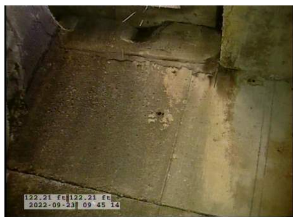
12, 00:06:26, 122.21ft Deposits Attached Encrustation, 5% of cross sectional area from 5 o'clock to 7 o'clock, within 8 inch, Finish / RUST
