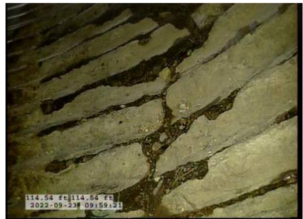
12, 00:06:50, 114.54ft Miscellaneous General Photograph from 5 o'clock to 7 o'clock / BOTTOM OF PIPE RUSTING AWAY
