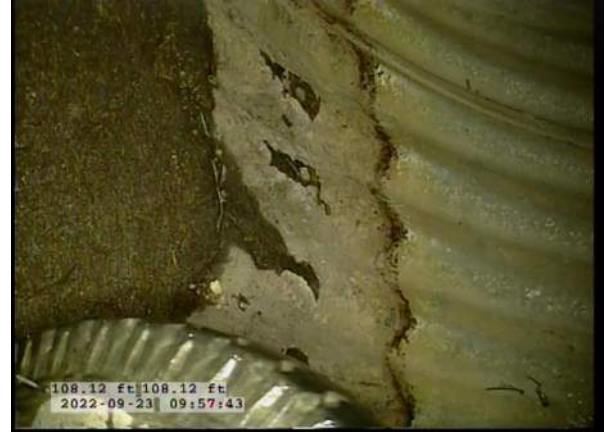
10, 00:05:42, 108.12ft Surface Damage Missing Wall from 5 o'clock to 7 o'clock, within 8 inch, Start / BOTTOM OF PIPE STARTING TO RUST AWAY, SMALL HOLES FORMING
