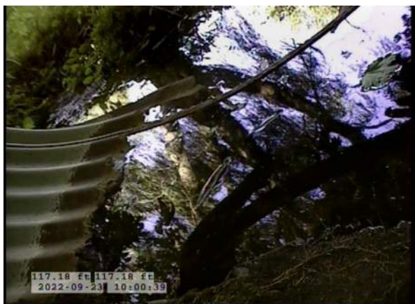
15, 00:07:26, 117.17ft Miscellaneous General Photograph from 5 o'clock to 7 o'clock / BOTTOM OF PIPE COMPLETELY MISSING AT END OF PIPE
