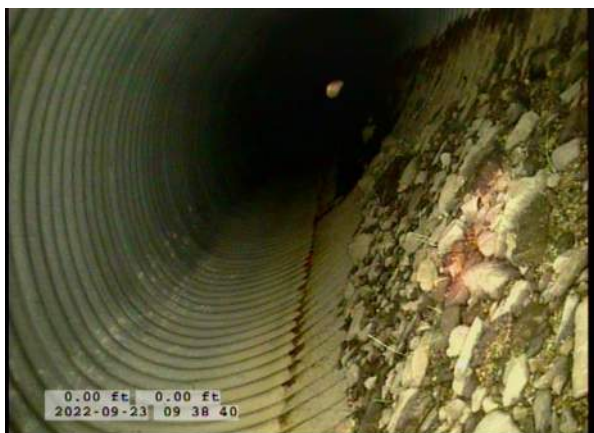
5, 00:00:34, 0.00ft Deposits Attached Encrustation, 5% of cross sectional area from 5 o'clock to 7 o'clock, within 8 inch, Start / RUST
