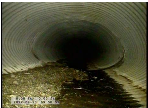
1, 00:00:10, 0.00ft Catch Basin / CB11
