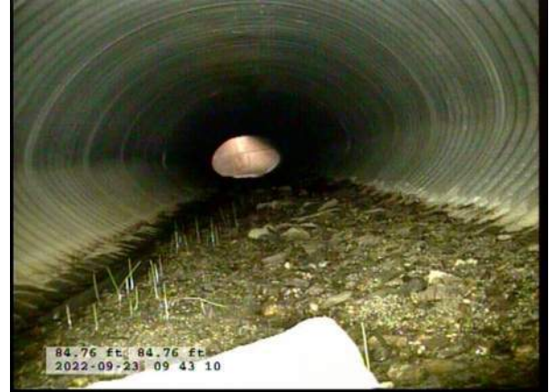
10, 00:04:32, 84.76ft Deposits Settled Gravel, 5% of cross sectional area from 5 o'clock to 7 o'clock, within 8 inch, Start
