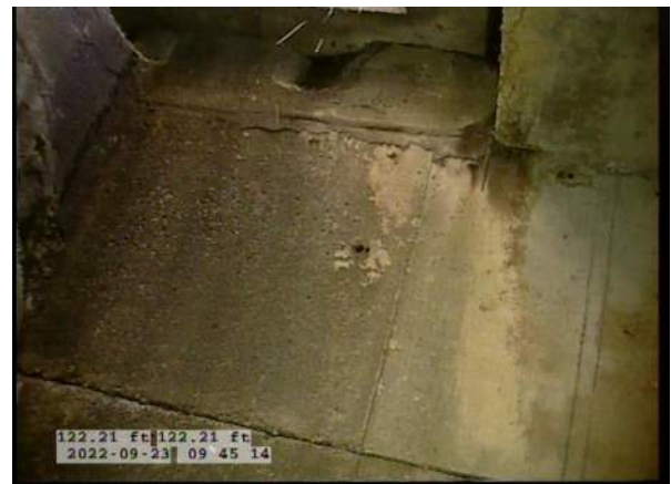
12, 00:06:26, 122.21ft Deposits Attached Encrustation, 5% of cross sectional area from 5 o'clock to 7 o'clock, within 8 inch, Finish / RUST
