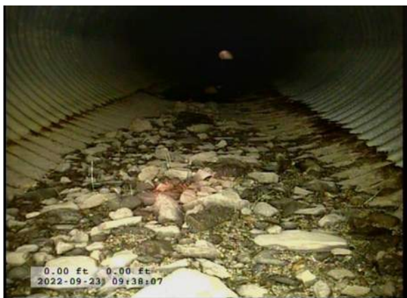
3, 00:00:24, 0.00ft Deposits Settled Gravel, 5% of cross sectional area at 6 o'clock, within 8 inch, Start
