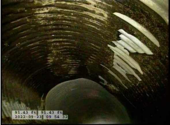
9, 00:03:14, 91.43ft Miscellaneous General Observation / BITUMINOUS COATING ON THIS LENGTH OF THE PIPE
