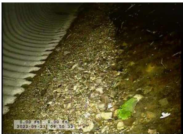
3, 00:00:24, 0.00ft Deposits Settled Compacted, 5% of cross sectional area from 6 o'clock to 7 o'clock, within 8 inch, Start
