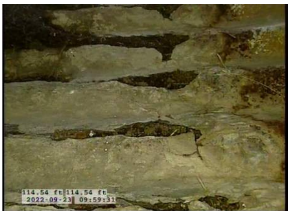
13, 00:06:50, 114.54ft Miscellaneous General Photograph from 5 o'clock to 7 o'clock / BOTTOM OF PIPE RUSTING AWAY
